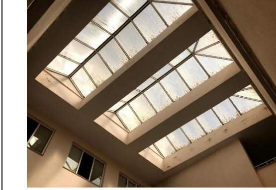
Transparent roofs for natural daylight lighting
