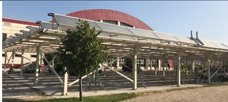
Solar absorption for heating the water used in school of medicine and swimming pool
