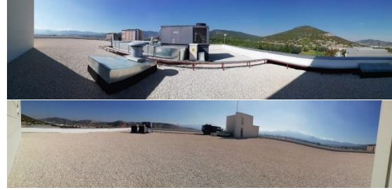
Example of roofs for new buildings (Early stage of constructing green roof)
